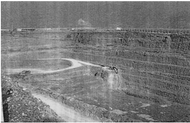
Fig. 5 View of the gravel pit between the ramblas of Bernal and VÍcar. The machine in the distance gives an idea of scale
